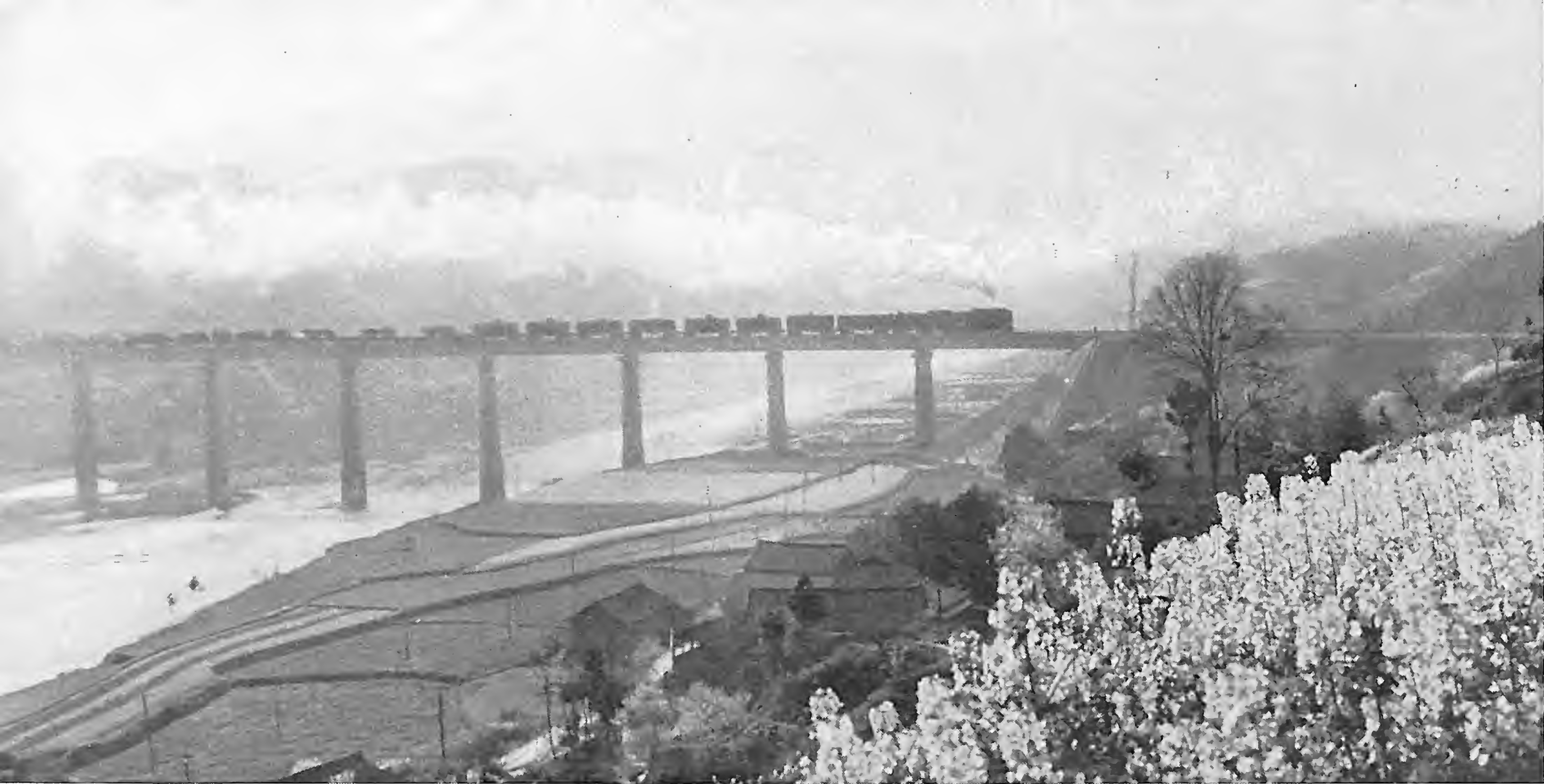
A freight train on the new line.
